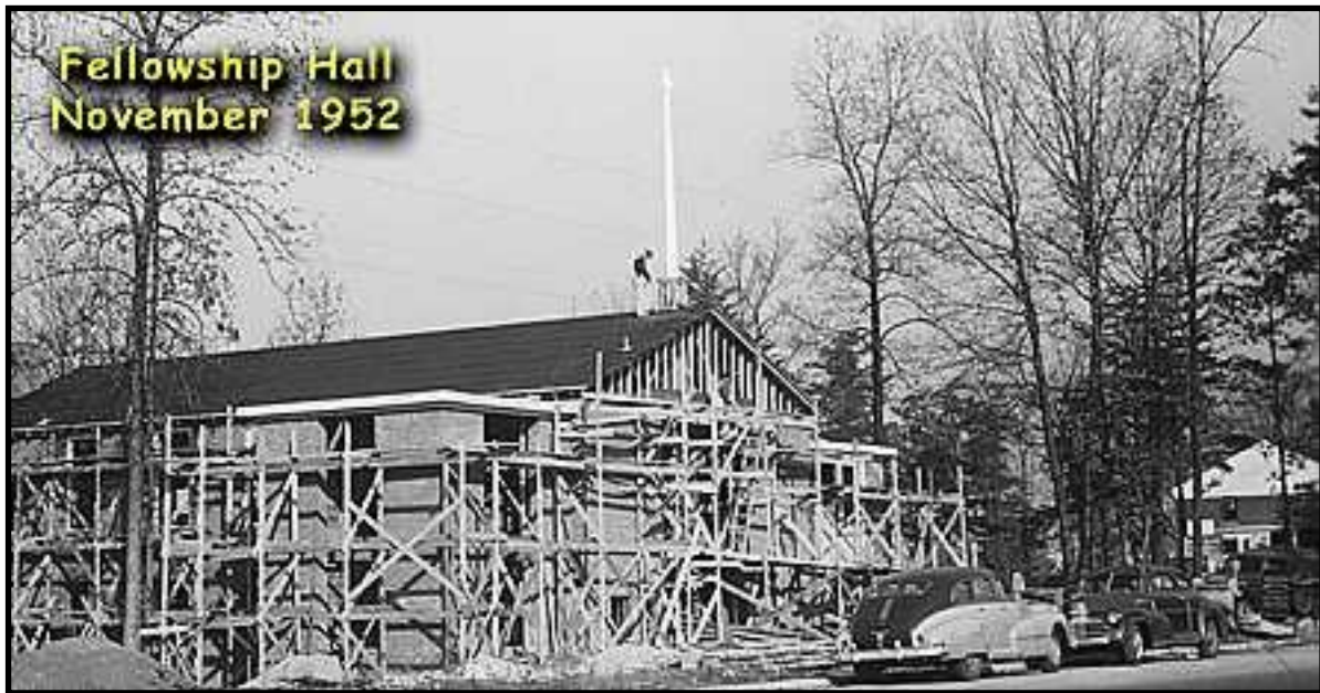
Knox Presbyterian Church under construction.
