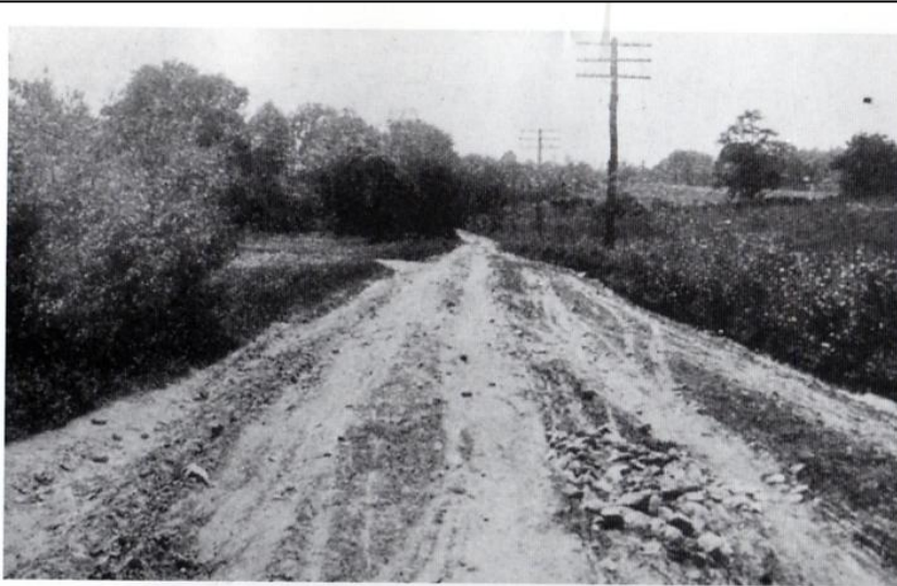
Lee Highway between Falls Church and Fairfax Court House, circa 1923. The dirt road, despised by many as a seasonal mud wallow, was selected to carry the designation Lee Highway, a newly-established route crossing the country from coast to coast. It was very difficult to drive anywhere, and unified routes such as this one bearing but one name proved so popular they were later numbered. Courtesy Mary Riley Styles Public Library.
