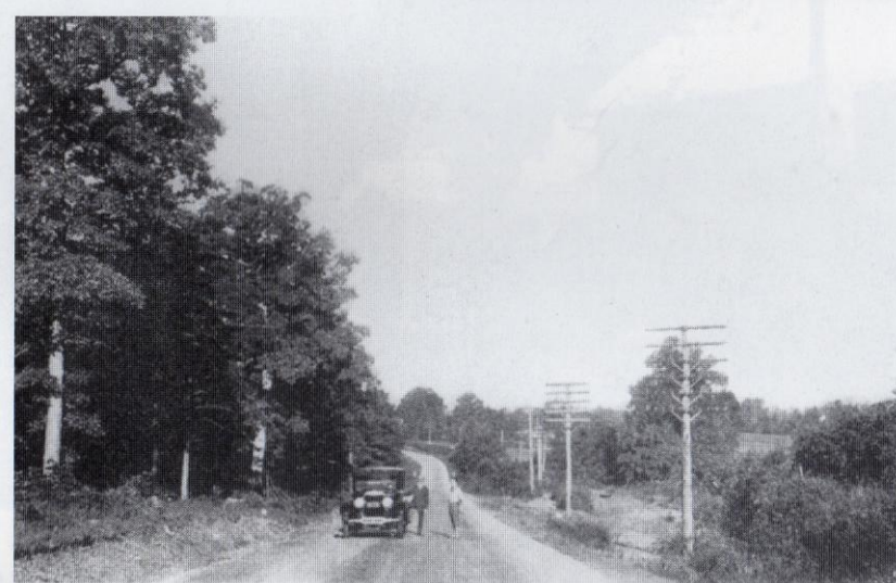
Lee Highway between Falls Church and Fairfax Court House, circa 1926. Falls Church businessman Merton E. Church, with foot on the automobile's running board, shows off the newly improved road, now eighteen feet wide and paved with concrete. The main trunk telephone line between Falls Church and Fairfax Court House, also built by Church, is seen at right. Courtesy Mary Riley Styles Public Library.
